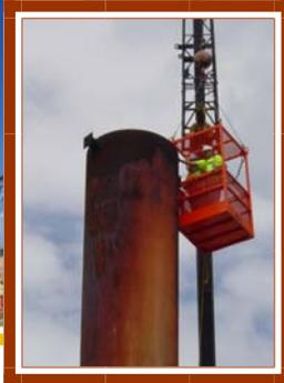
quite a challenge for our employees. The work began by hoisting a man up to the top of the stack in a man basket hooked to the crane to weld new picking hooks onto the steel extension. Once the picking devices were in place, a crane hooked onto the steel extension while another crane held onto the structure holding the extension in place as it was cut free by a man in a boom lift. Once the extension was cut free, the
