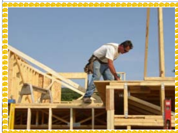
Picture: Curt Willson lending a hand at Habitat for Humanity
