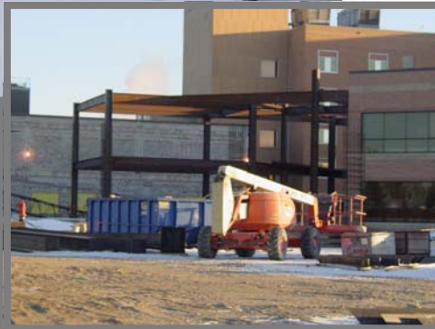
Right: Steel erection begins on the ISJ/MHS Cardiology Expansion.
