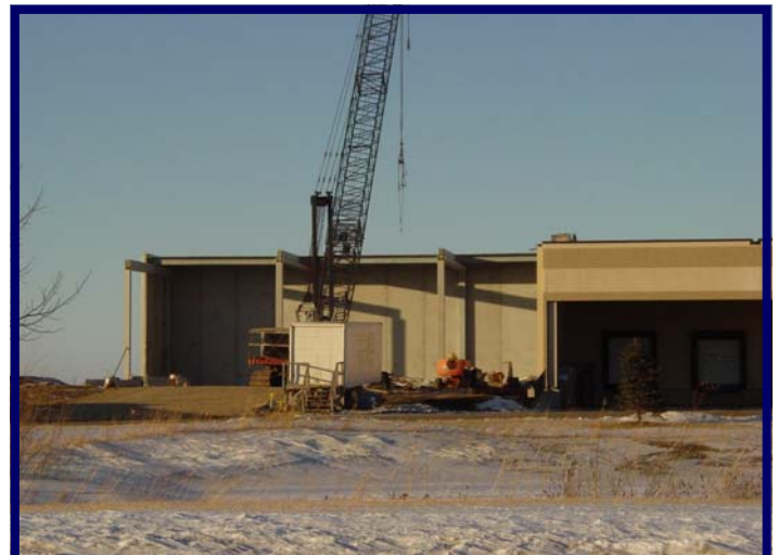
Pre-cast panels going up for the Label Works warehouse addition.
